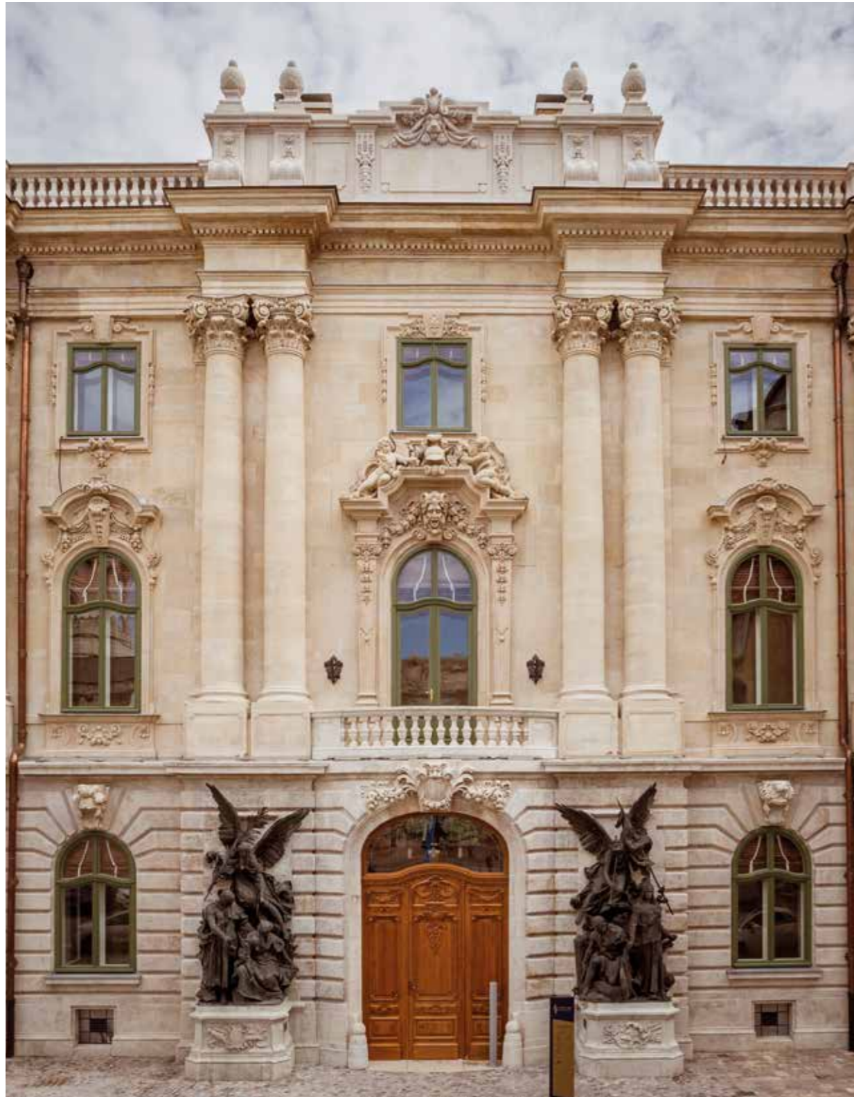
The north façade renewed, 2021
