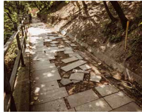
The Ellyps Promenade before renovation
