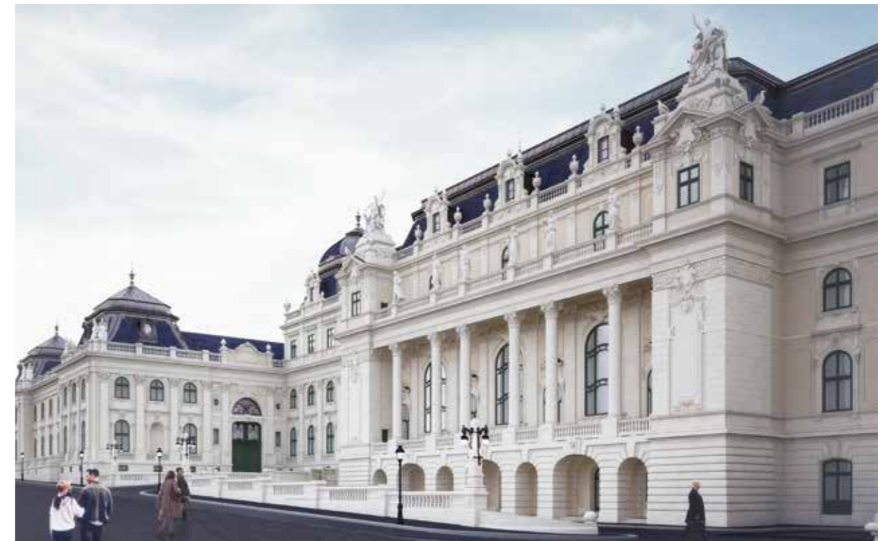
Visual designs of the north wing of the Palace of Buda Castle
