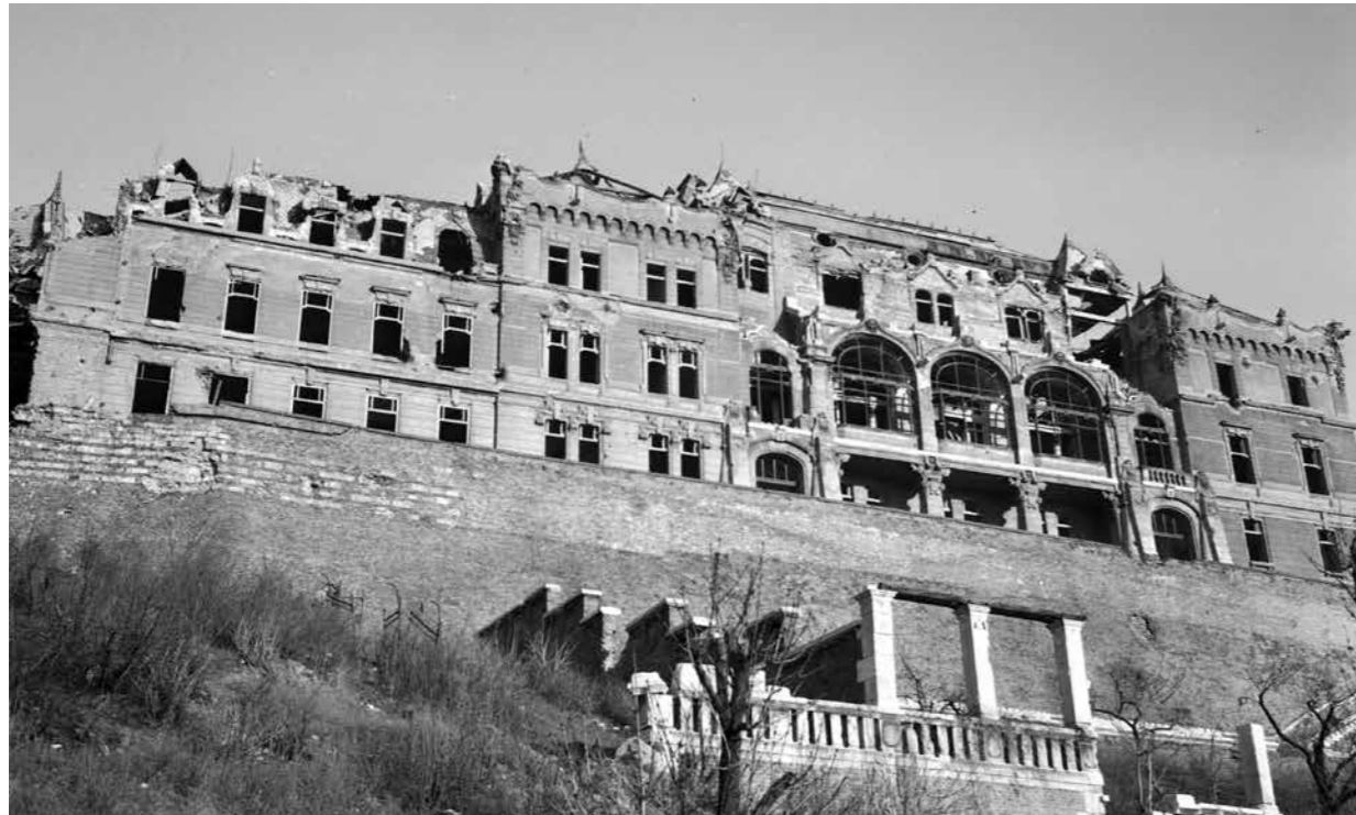
The building was damaged during the Second World War II, 1949
