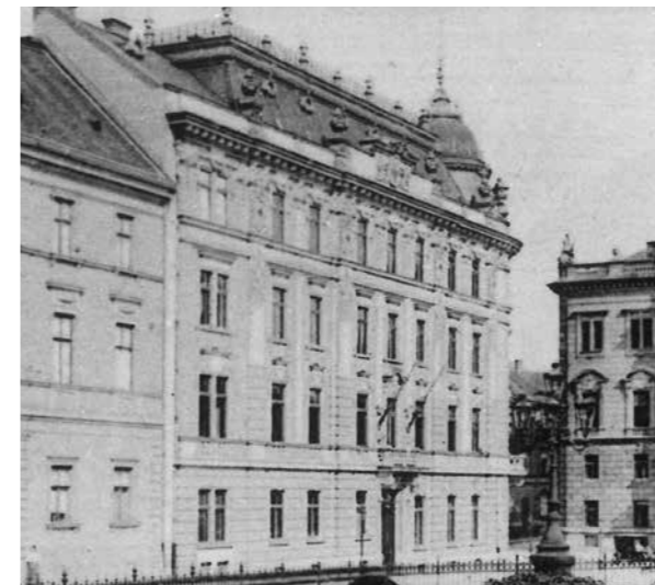
The western façade of the building around 1910
